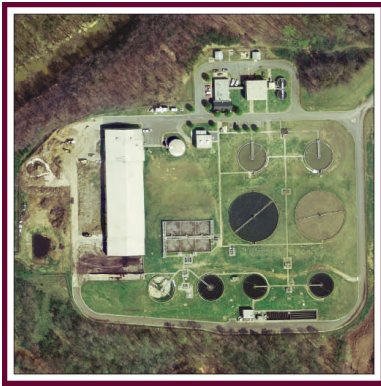
Aerial of First Broad WWTP
